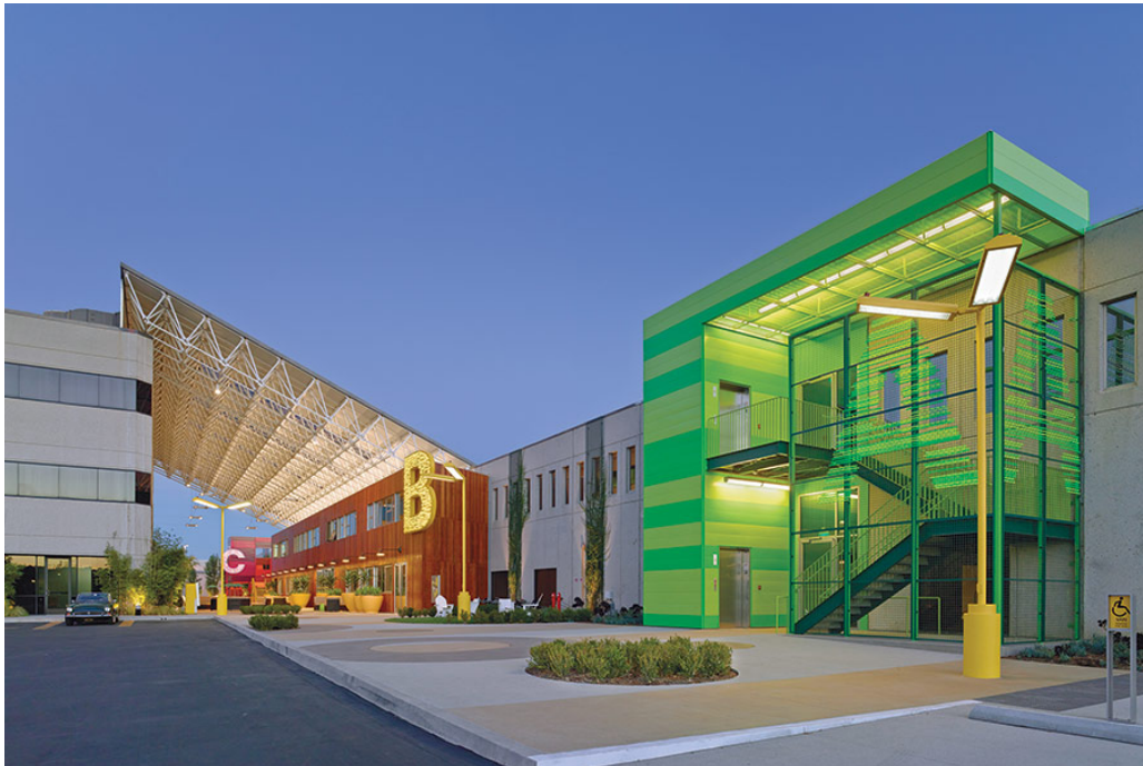
THE FIRM HAS CREATED A NEW ENTRY AND CONGREGATING AREA ON THE SITE OF A ONCE DARK AND ENCLOSED ATRIUM. FOTOWORKS
